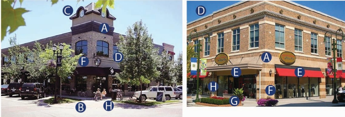
FIGURE 4. PRIMARY BUILDING ENTRANCES
